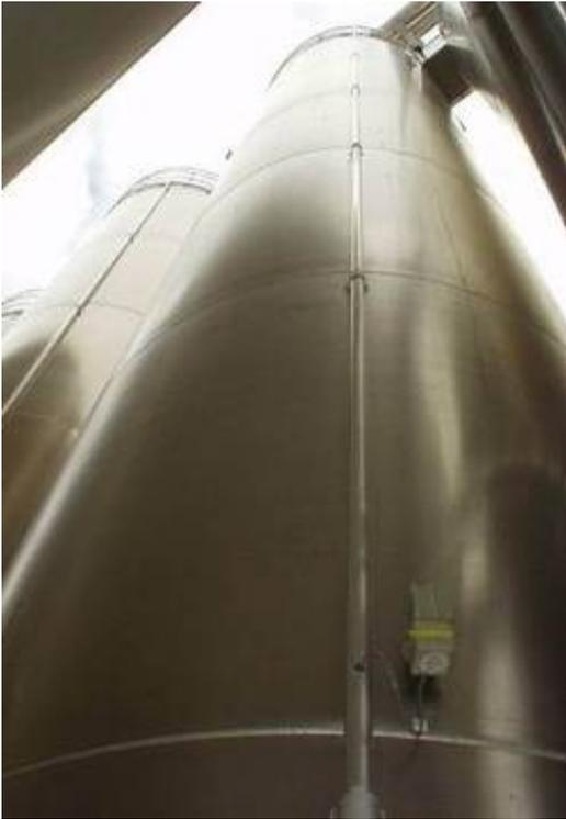
A German manufacturer of food packaging stores its plastic granules in a few double chamber silos. The challenge in this application is to measure the lower chamber through a long tube leading from the silo through the upper chamber. A non-contact sensor such as ultrasound or radar does not work reliably because the long tube attenuates the reflected signal or even leads to incorrect measurements by wrong echos.
